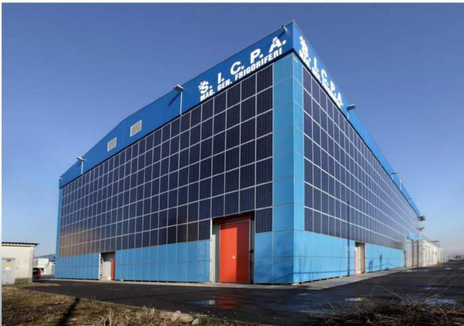
*The Omniablok system is also perfect for façade applications. The vertically-mounted framework allows installing photovoltaic panels at the centre and rolled aluminium sheet panels painted with epoxy powders along the perimeter. Thanks to this solution, the façade of the building is not affected by the intervention in question, neither structurally nor aesthetically.*
