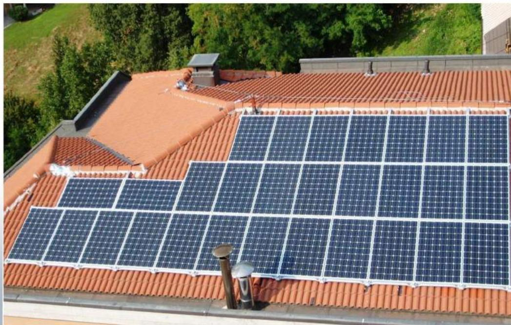
*The system in the photo extends on only one pitch of the roof and this requires providing at least one fastening point so as to guarantee the stability of the system. The Omniablok framework is constrained through a series of iron plates fastened to the ridge point of the roofing, where there is the least risk of infiltration. The body of the framework rests on the pitch without perforating it.*
